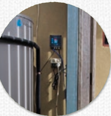
Reclaim Heat Pump Hot water system installation. Photo: Julian Higgs.
